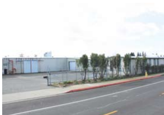
Large industrial/manufacturing property. Building is 51,500 SF on 5.5 acres of fenced and paved yard area. Building has 16-18 ft ceilings, oversized grade level doors, and 800 amp voltage. Call Greg Quilty (530) 632-8634.
